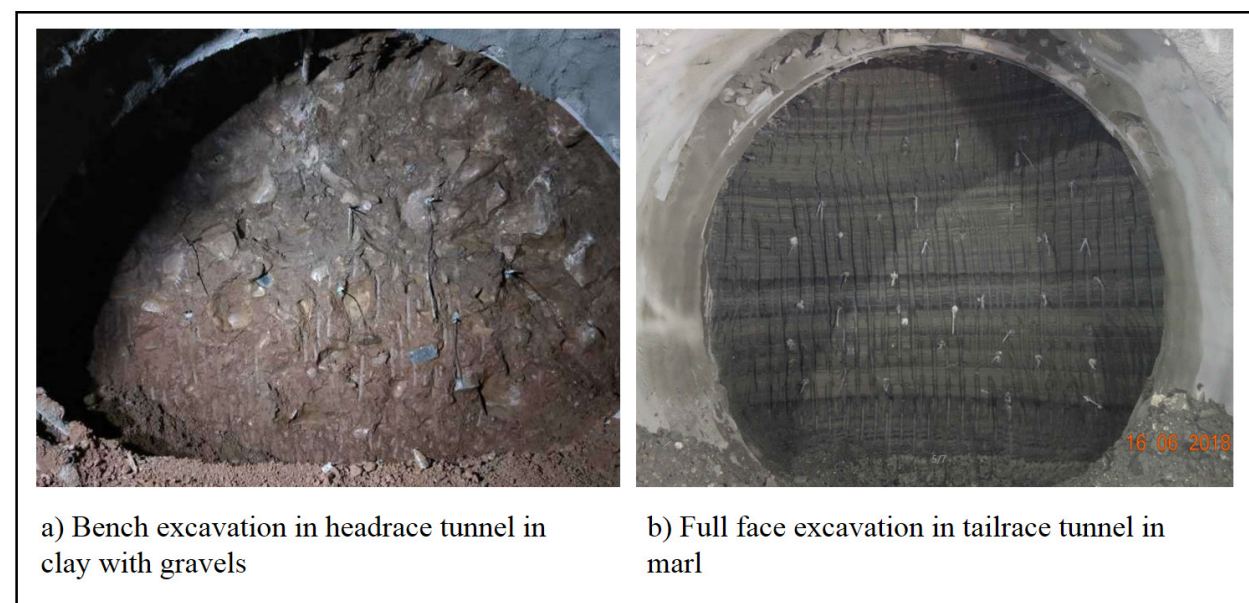
Figure 1. Photographs of the tunnel faces reinforced with fiberglass anchors.
